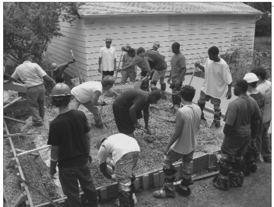
Grading the foundation
