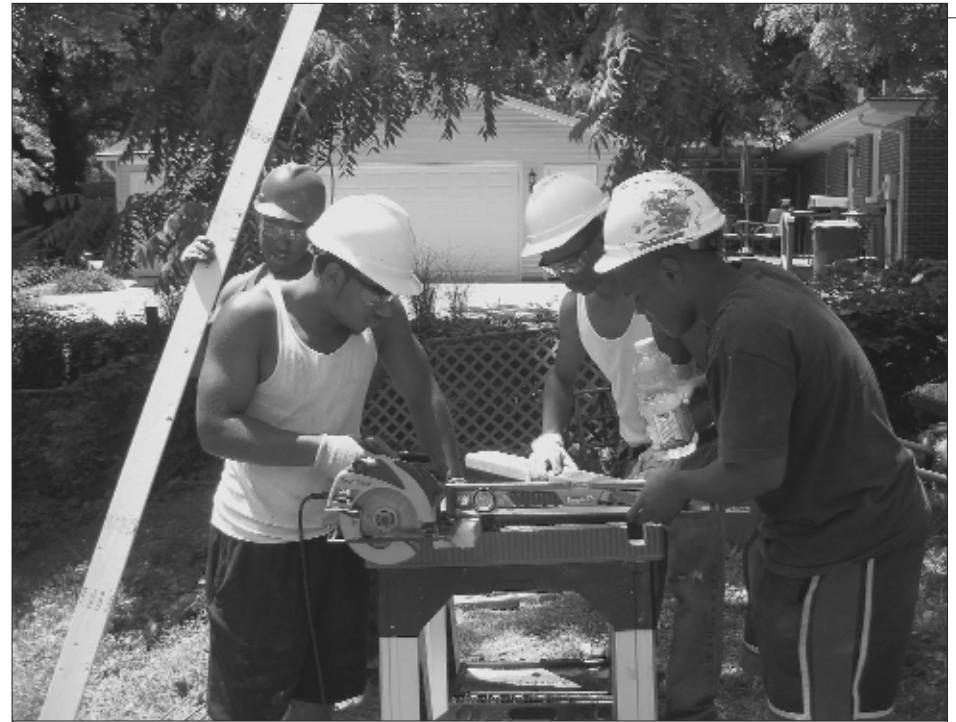
Learning cut boards for framing the garage
