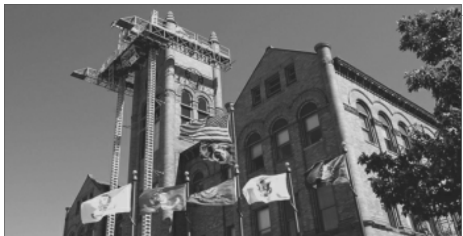
The Champaign County Court House clock tower restoration
